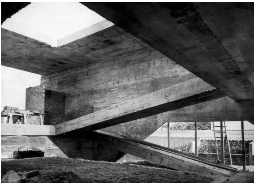
6. Bittencourt House, architects Artigas & Cascaldi, SP, 1959
