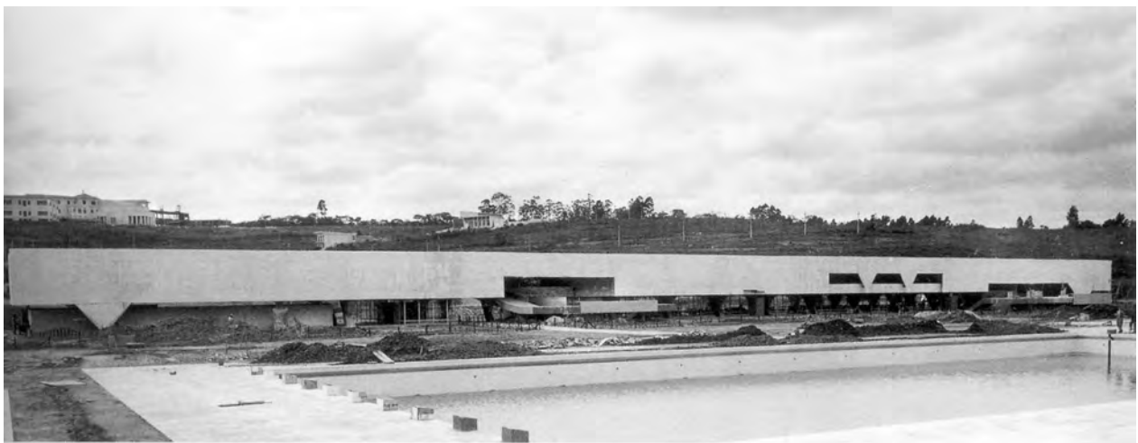
10. São Paulo Football Club Dressing-Rooms, architects Artigas & Cascaldi, SP, 1961
